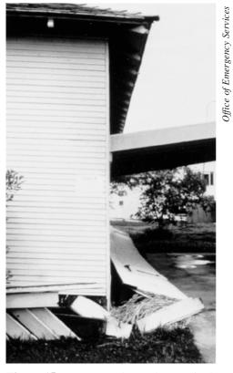
**Figure 15** - Damage to home due to cripple wall failure.
