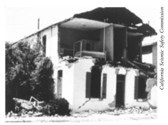
**Figure 25** - The plaster-covered brick walls of this building collapsed during a recent earthquake.
