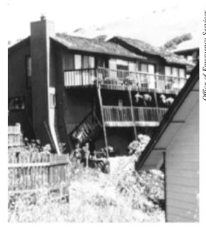
Figure 22 - This hillside home was built on an unbraced tall wall that failed.
