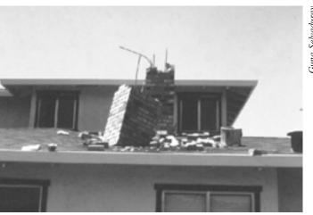
Figure 34 - Morgan Hill Earthquake. Broken chimney fell on
