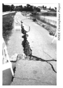
**Figure 39 - Lateral Spreading.** Loma Prieta Earthquake, October 17, 1989. Lateral spreading damage levee road along the San Lorenzo River.
