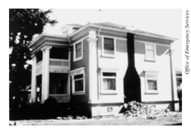
Figure 33 - This unreinforced chimney fell during a recent earthquake.
