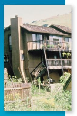
The balcony of this hillside home partially collapsed and the home tilted when the stilt-type support posts and poorly braced walls shifted during an earthquake.
