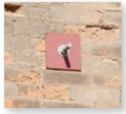
A steel plate with anchor bolts.
